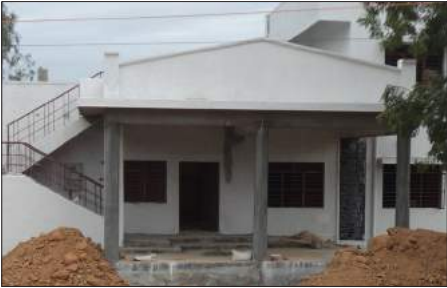
The construction of police station at Avalahalli is nearing completion
