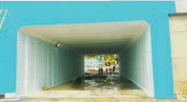
Uturn Push box underpass under Marathahalli bridge
